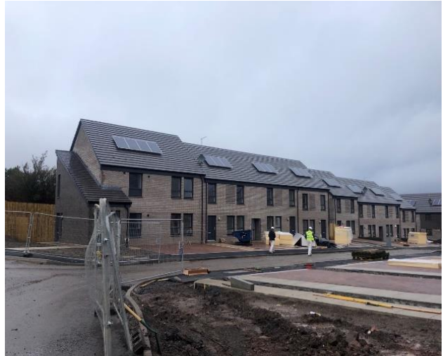
Oak Tree's Tweed Street site in development, Greenock
