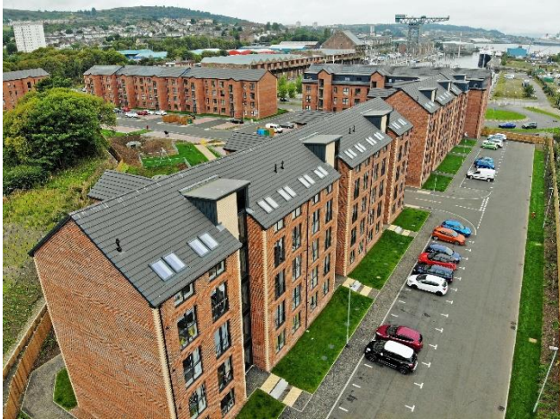
River Clyde Homes' James Watt Dock development, Greenock
