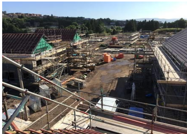
Link's Ravenscraig site in development, Greenock
